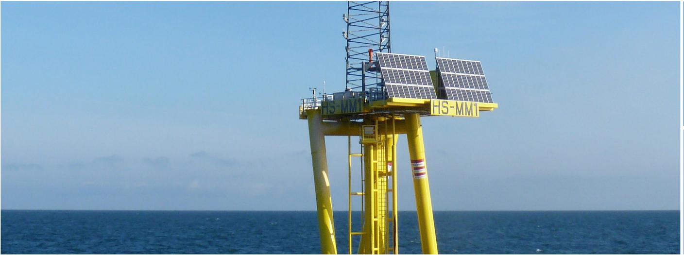
**RES Offshore offers met' mast design, supply, installation and AO&M (Asset Operation and Management) services for offshore project developers, both on a turnkey and a project management basis, together with metocean data collection systems and data analysis.**
