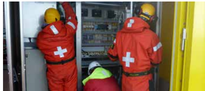
Replacing and Calibrating Equipment
